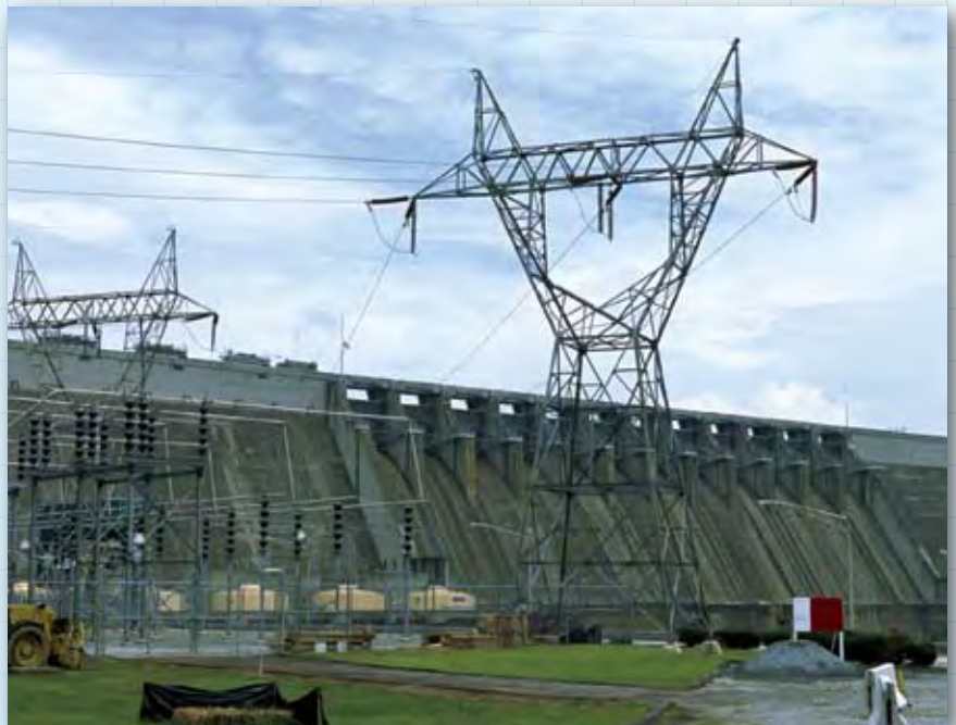
This power plant in Tennessee uses hydroelectric energy to produce electricity.
